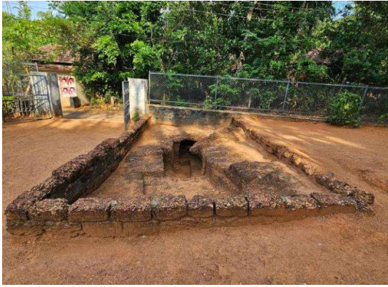
Image 1: Approach road to the monument
