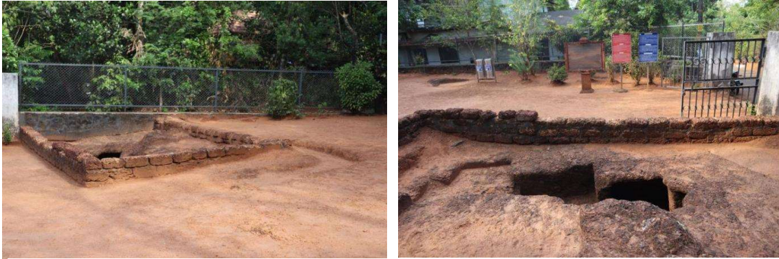
Image 6: Views of the temporary drains on site and open roof of monument
