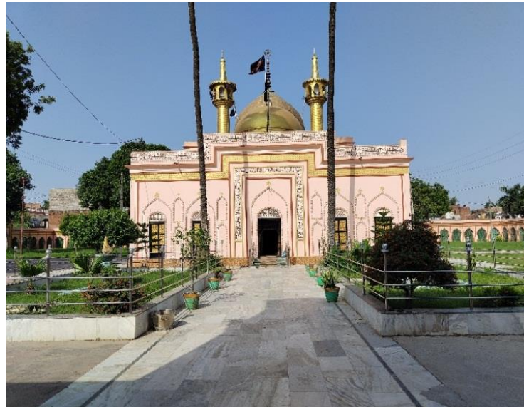
Fig 13. A dilapidated heritage structure along with protected monument of Karbala of Dainut-ud Daula.in west direction
