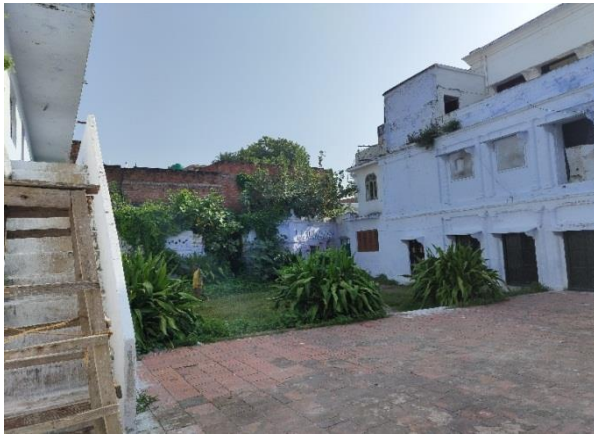
Fig 7. Kothi Agha Abu Khan ka hatta in south-east direction
