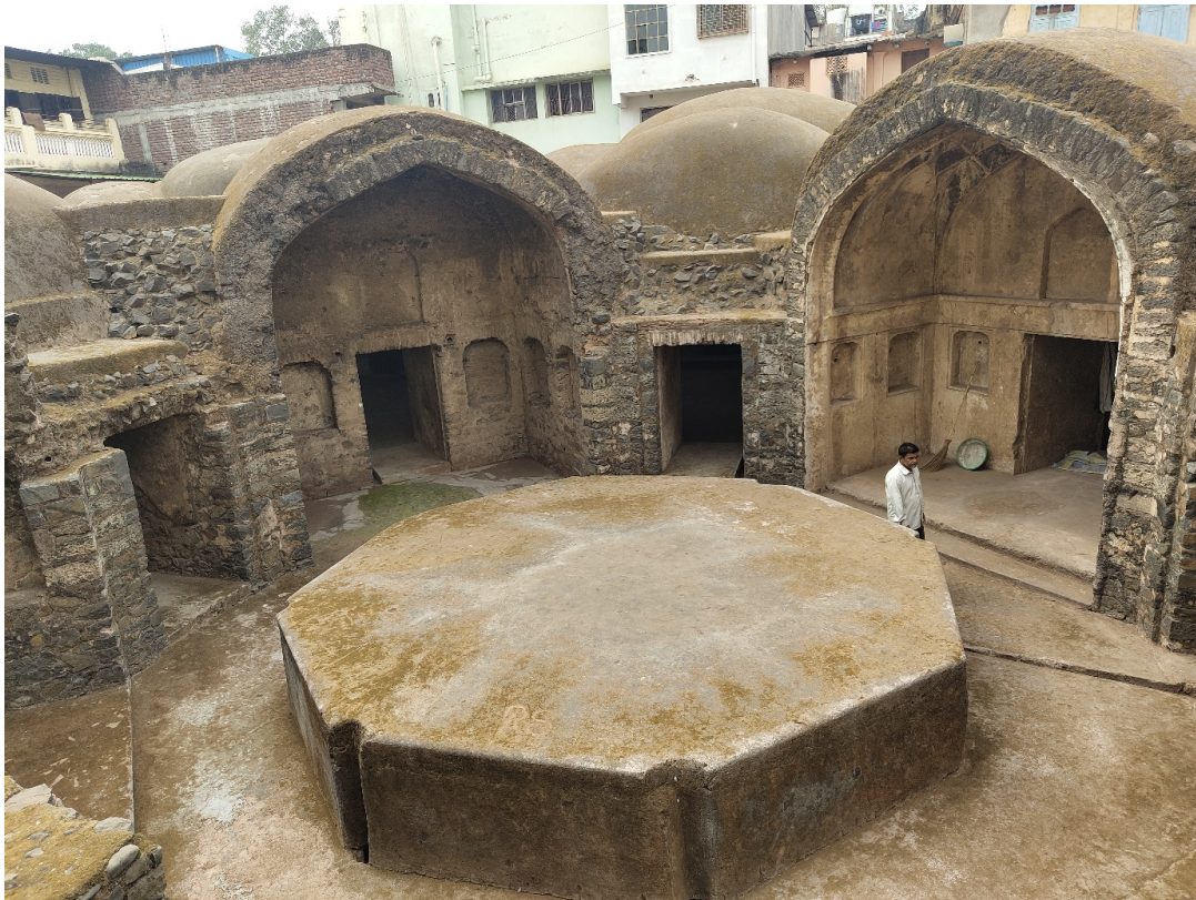
Figure 8: Existing Condition of Monument- 2
