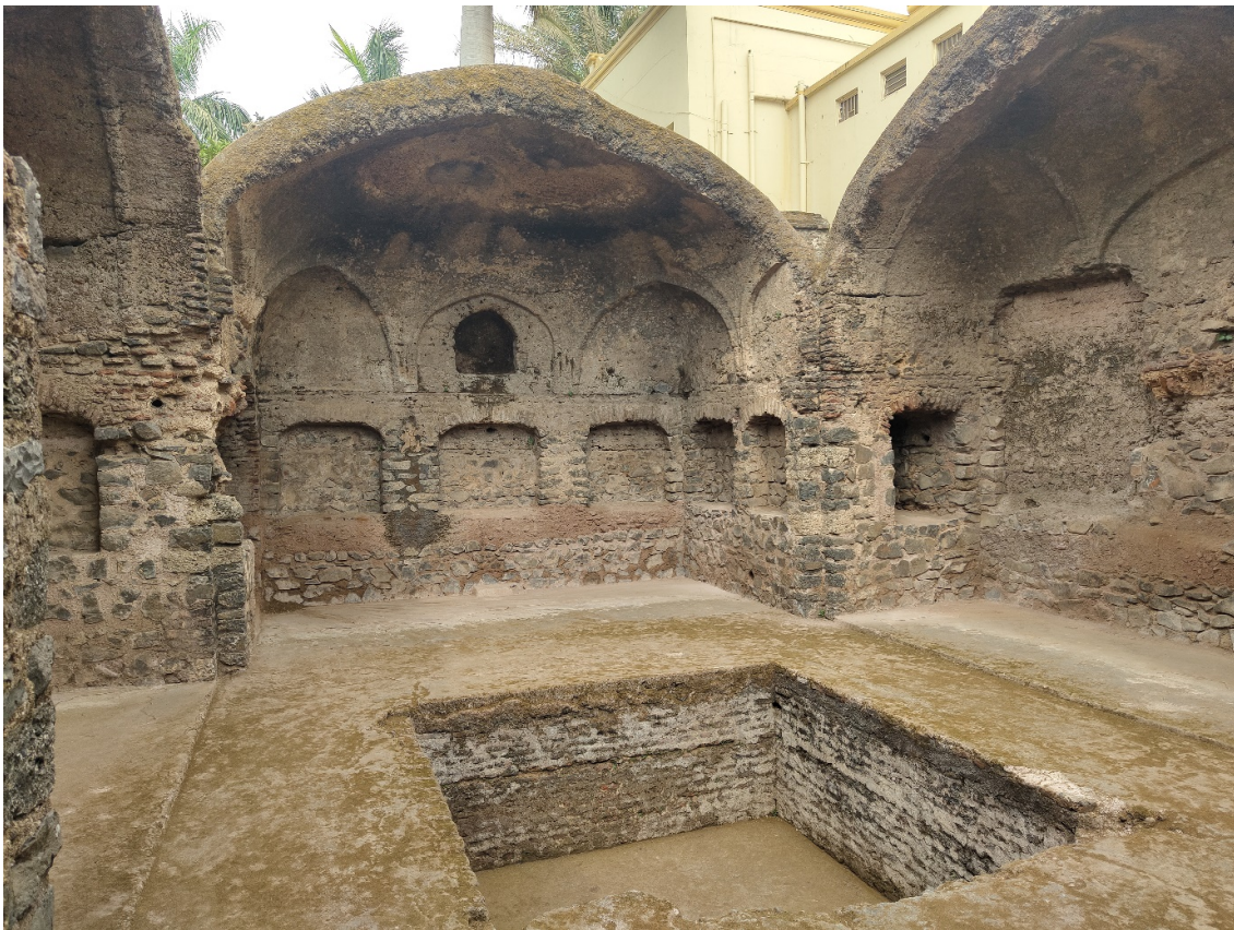
Figure 10: Existing Condition of Monument- 4
