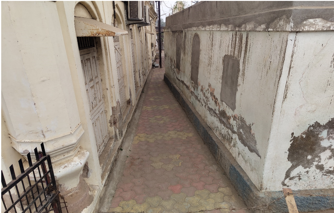
Figure4: Approach Road/Gali to Hammam Khana
