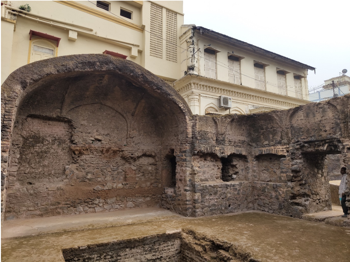
Figure 9: Existing Condition of Monument- 3
