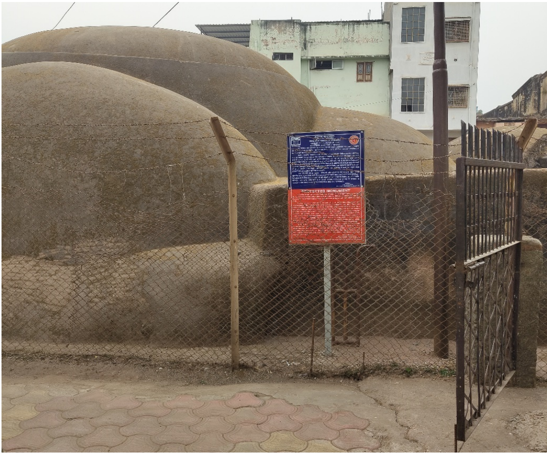
Figure3: Entry Gate to Hammam Khana
