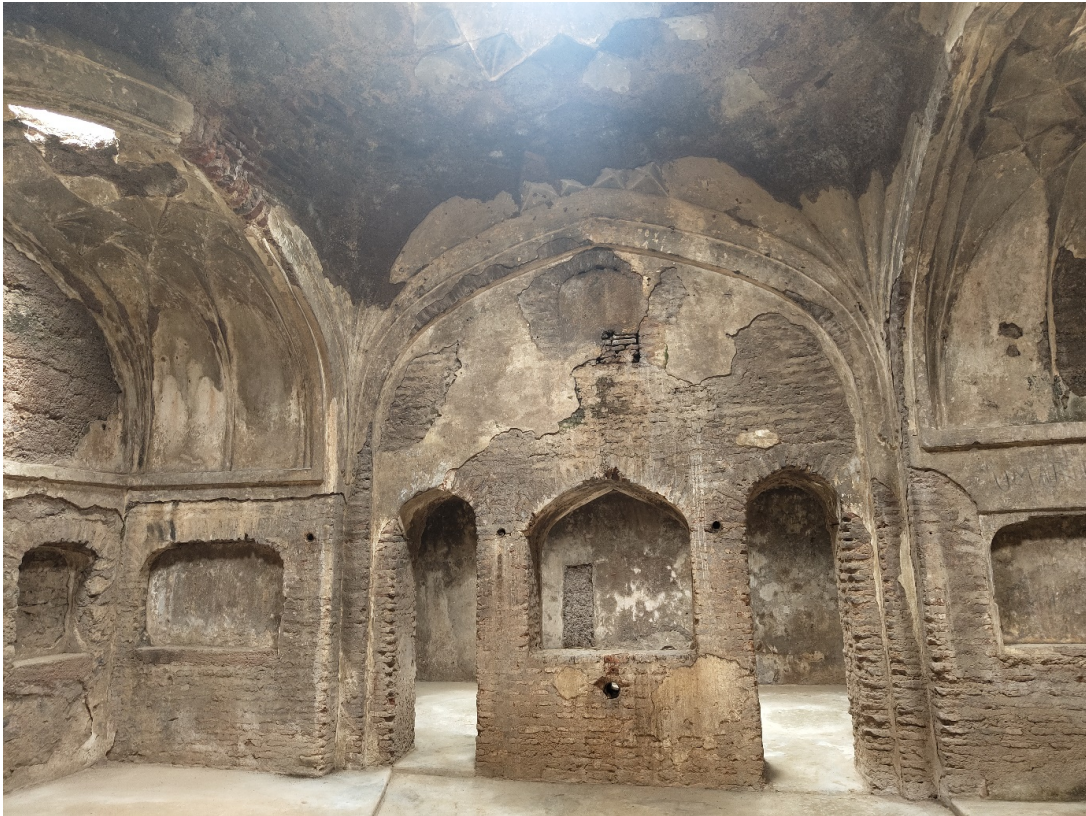
Figure 7: Existing Condition of Monument- 1
